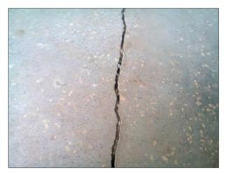
Plate 5 Cracked Floor Slab; Source: Researchers field study (2018)
