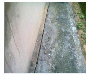
Plate 2 Crack and Dampness at the Foundation ; Source: Researchers field study (2018)
