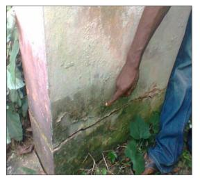
**Plate 1** Longitudinal Crack and Dampness at the Foundation; Source: Researchers field study (2018)
