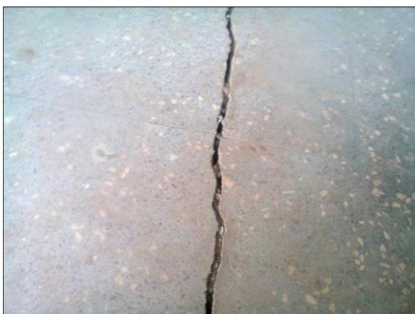
**Plate 5** Cracked Floor Slab; Source: Researchers field study (2018)
